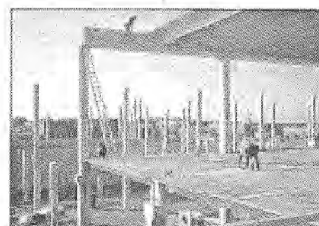
Figures 6a and b: Parallel presentation of composite sketch assembly with site photo showing the actual installation of the element.
