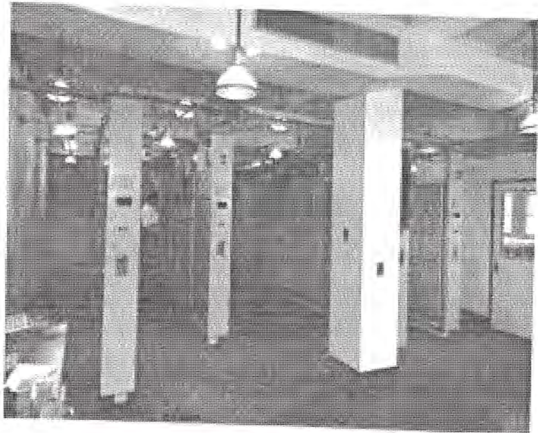
Figure 1. U.S. Army Photo A51244. Bell Relay Computer, showing racks in which the computing, storing and controlling relays are mounted.
